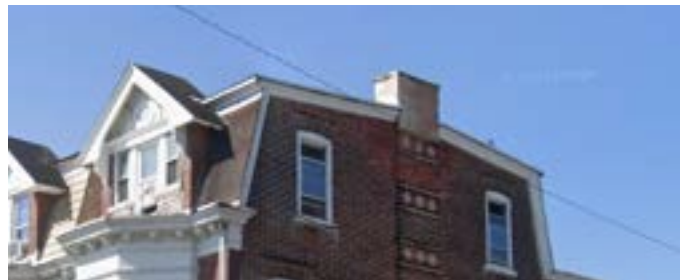
Pitched Roof Type (Gambrel Roof)
