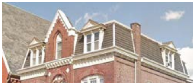
Pitched Roof Type (Mansard Roof)
